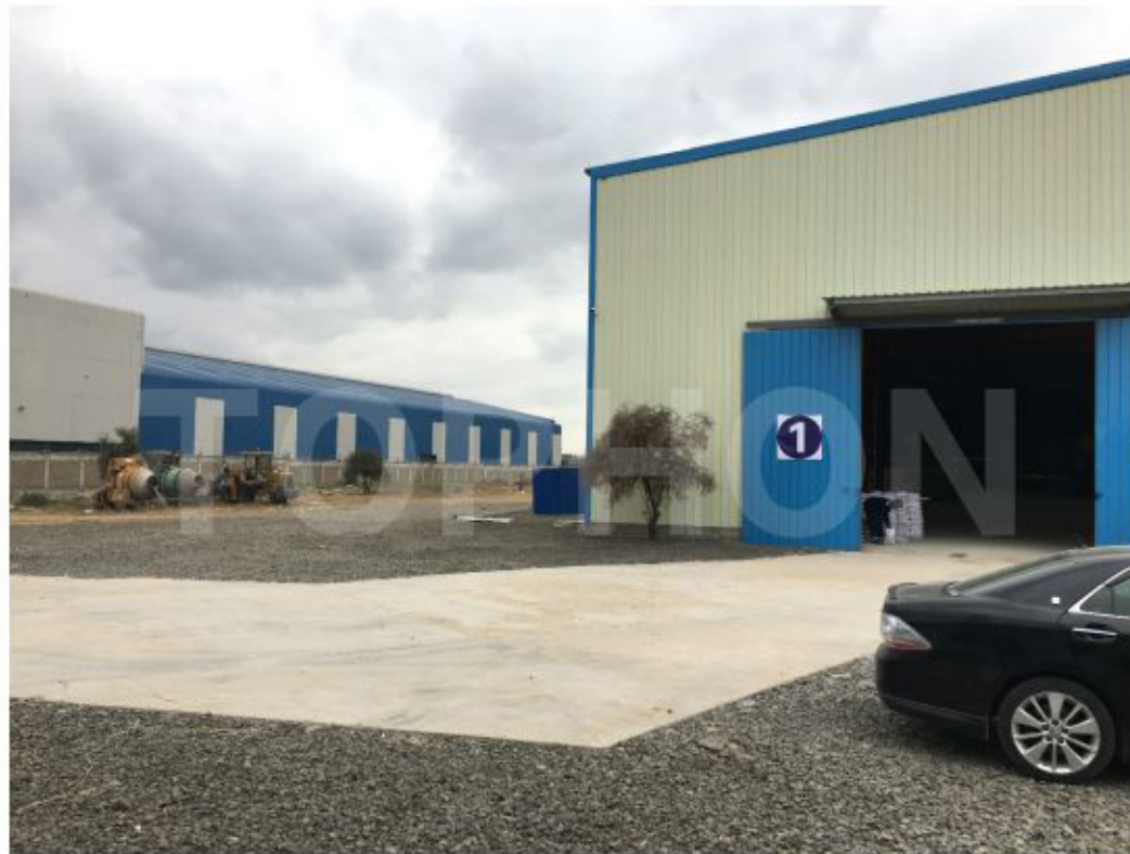
Overview picture of local factory
